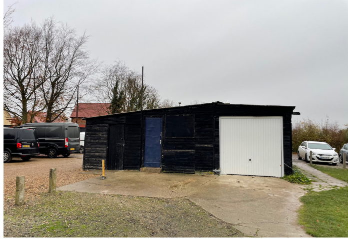
Existing northern shed
