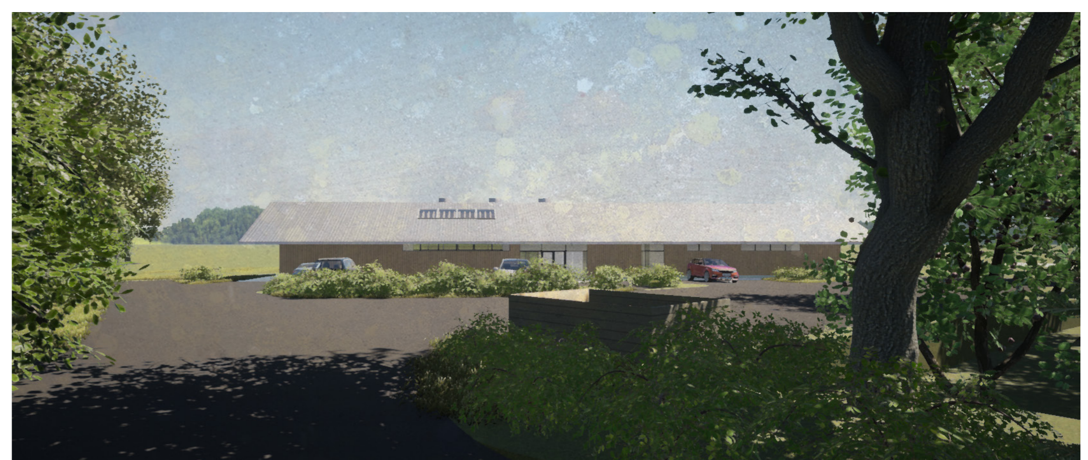
Approach to Building
