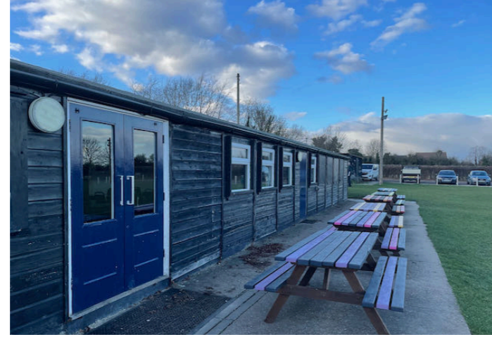
Existing eastern side with seating area
